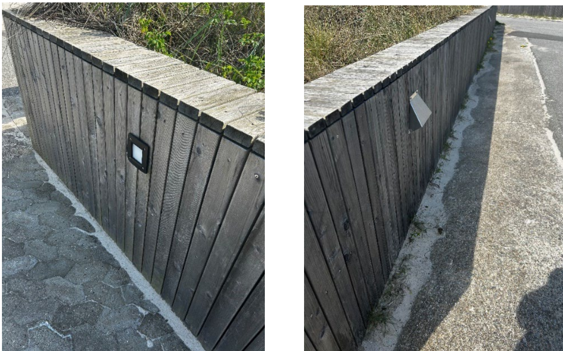
Figure 7.2.C. Barbecue area at Anholt Harbor. Examples of non-shielded lighting (at left; 2023) and with dark-sky friendly shielded lighting (at right; 2024). By year-end 2025, all these lights will be shielded.
